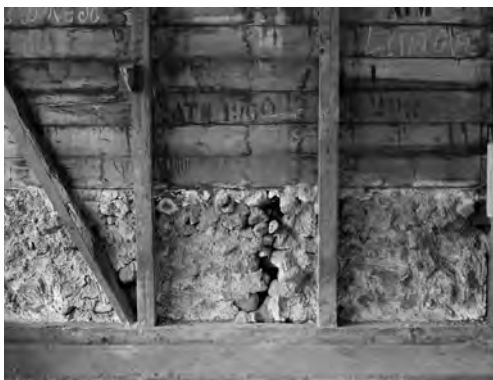
Figure 7: Vaitea Farm Shearing Shed in 2017 surrounded by Eucalyptus trees; the former wool press housing and timber lined walls, with brand marks, above the concrete base wall (photos by author).
